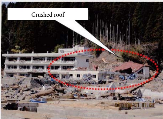
Badly damaged gymnasium
