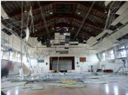
Fallen ceiling material and lighting fittings
