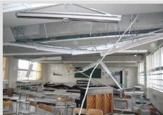
Fallen ceiling material and lighting fittings
