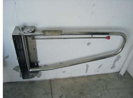
A swing type handrail in the renovation plan at the beginning
